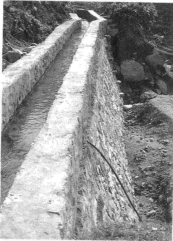
Photograph 8A Cement Masonry Retaining Wall to Support a Lined Canal
